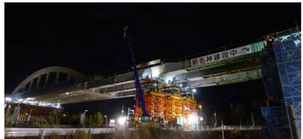
Fig. 7: The 'one-night' bent
