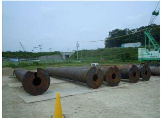
Fig. 5: Screw steel pipe piles with toe wings
