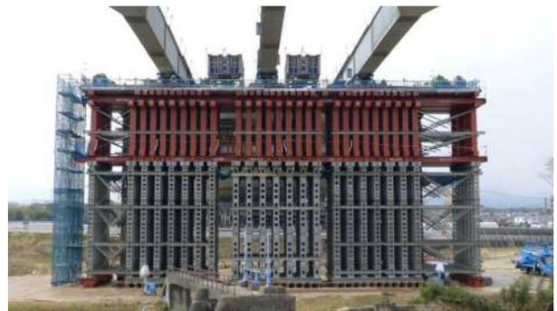
Fig. 8: Bent positioned in the river
